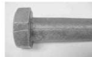
FIGURE 2.08 Crack in bolt
