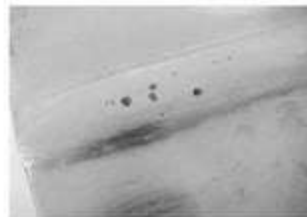
FIGURE 2.04 Surface porosity in weld
