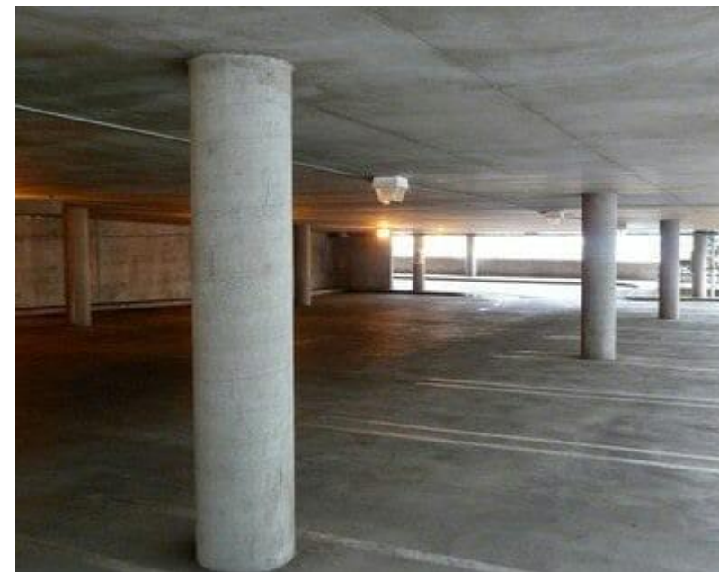
Flat plate floor system
