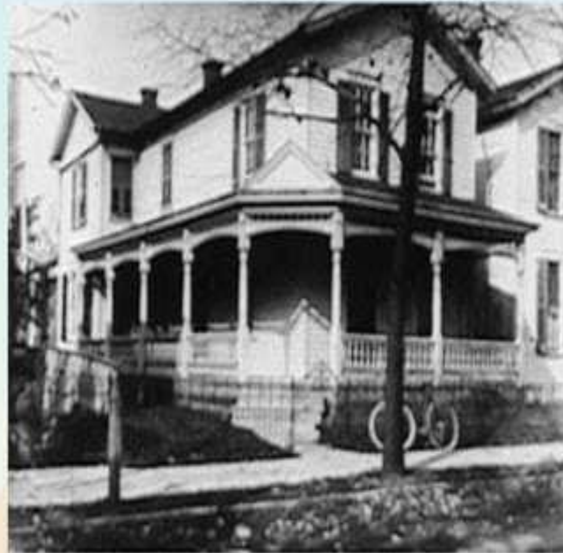
The Wright House, 7 Hawthorne Street , Dayton, Ohio
